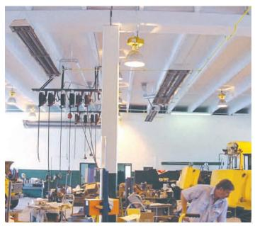
A highly radiant efficient Space-Ray infrared heating system can normally save a building owner 30% to 50% in annual fuel costs compared to forced air heating systems.
